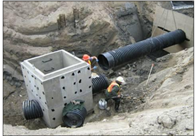
Figure 4. Installing a new 3-way water control structure at Leach Lake, October 2009. Photo by Marc-André. Beaucher.
