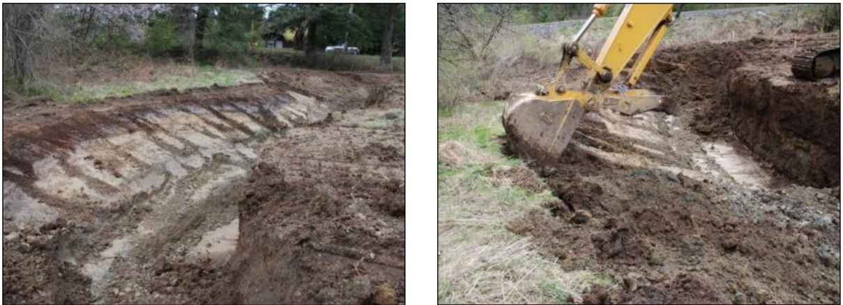
Figure 1. Creating a stream channel. Nature does not make a smooth surface; have your excavator operator create a slope that is loose and rough. Photos by David Polster.
