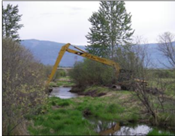
Figure 5. Dredging a channel in the Corn Creek Marsh.
