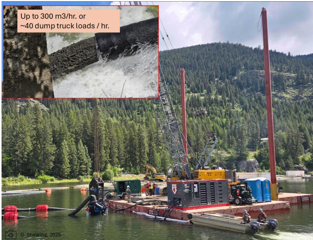
Figure 2. Active dredging in Spring 2025 at Wilsey Dam
