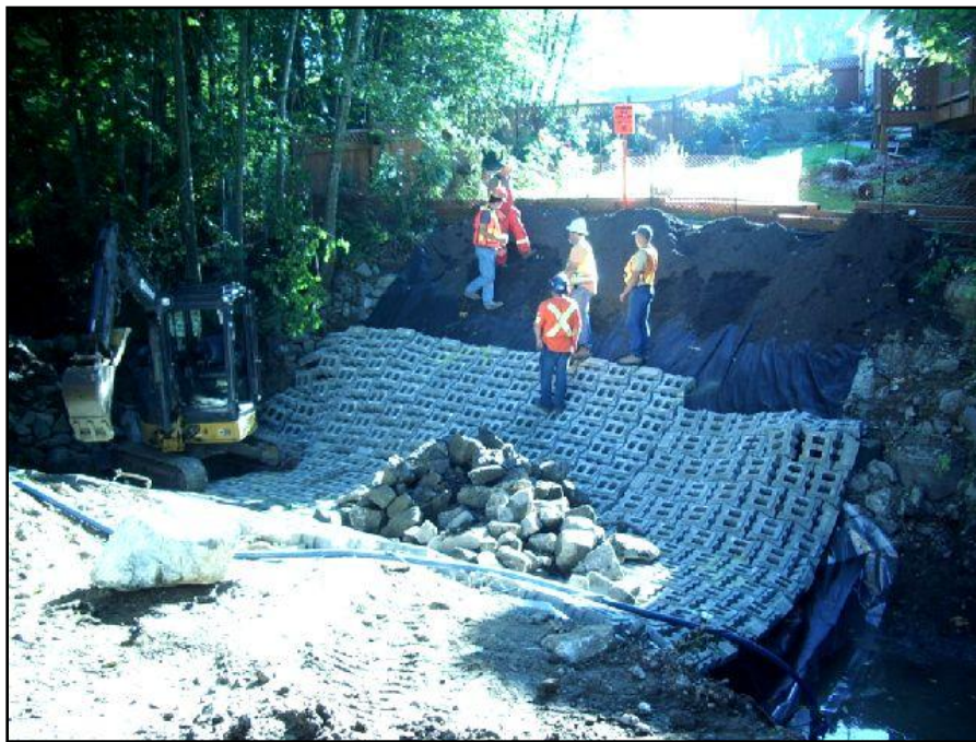
Figure 5. Mat placement at Cub Creek. The downstream excavation (photo right) is for keying mats to the channel bed and installation of rock riffles. These measures were necessary due to the high gradient and design velocities at this site.
