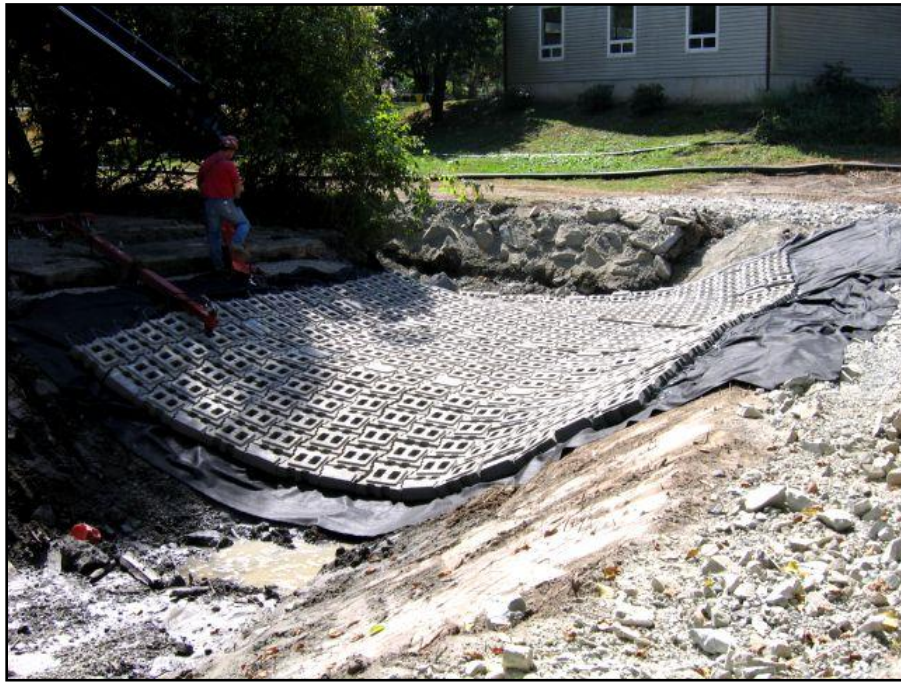
Figure 3. Mat placement at Nicomekl River crossing. Note that the channel cross-section is contoured so that low flows are concentrated near the left bank (photo right).
