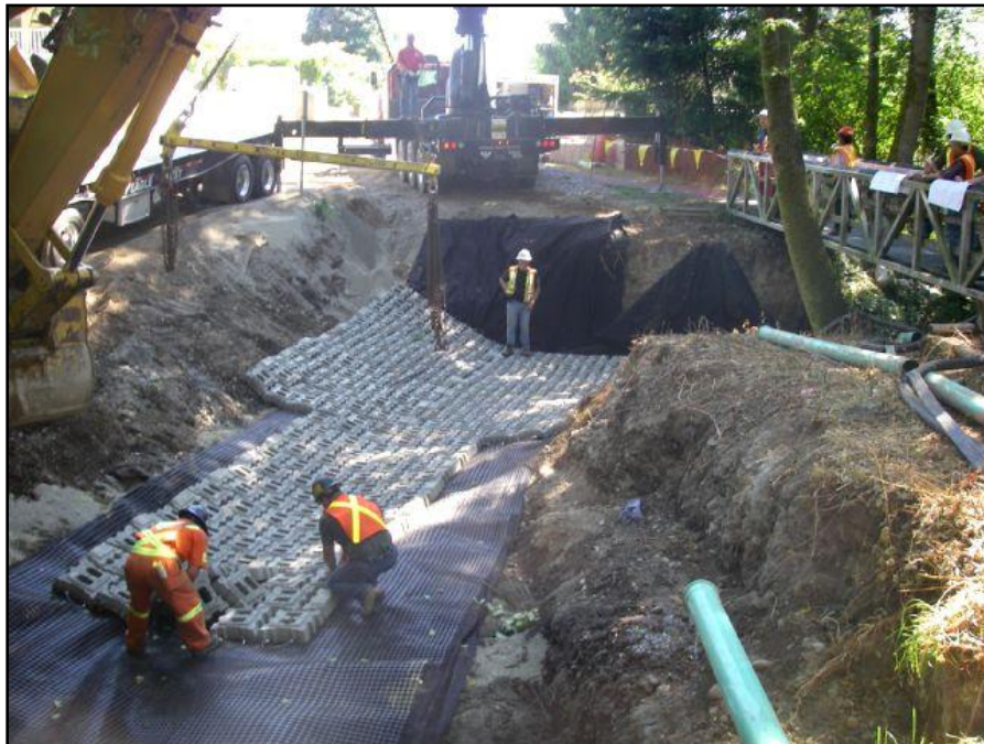
Figure 7. Mat placement at Price Creek.
