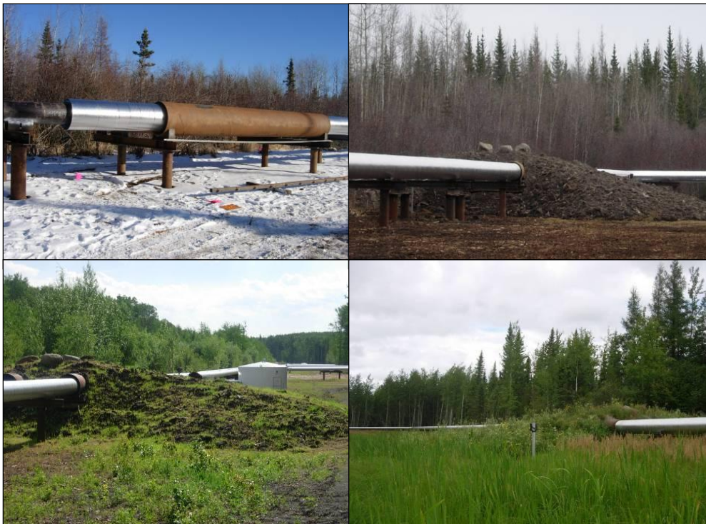
Figure 1: Construction of earthen pipeline crossing structures.
