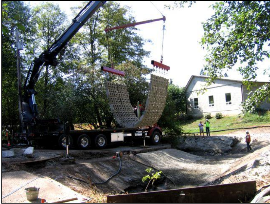
Figure 1. Typical concrete mat installation in progress. Generally, the amount of instream excavation can be reduced since keying mats to the channel bed is optional, due to the lower profile of mats compared to riprap
