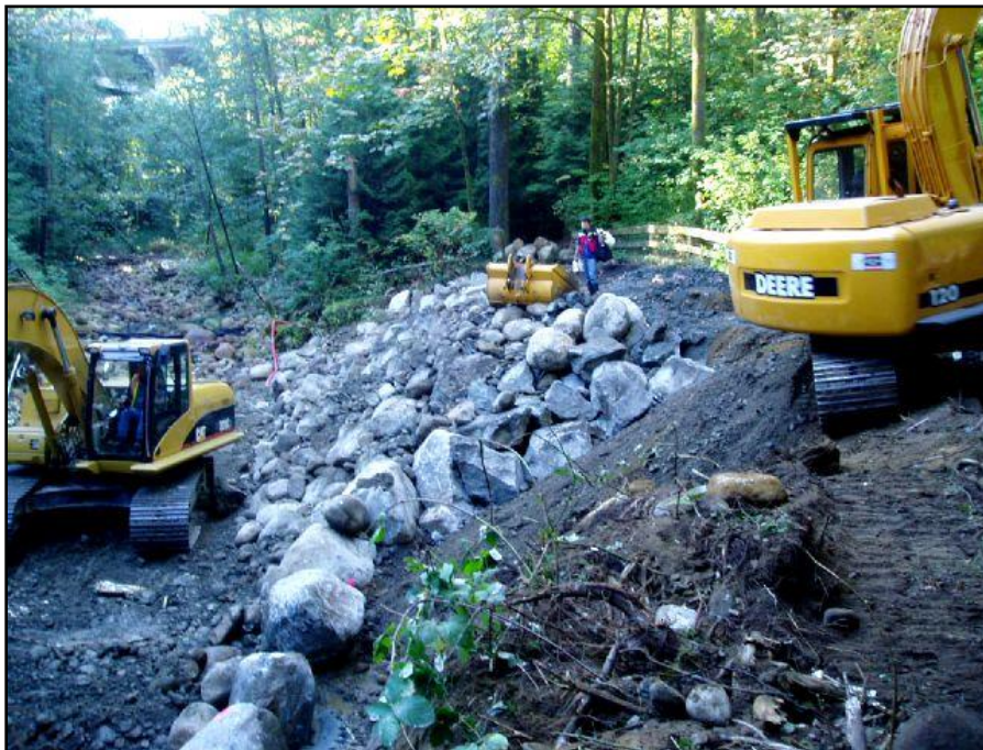
Figure 2. Typical riprap bank protection installation in progress. Riprap installations generally require extensive instream excavation.
